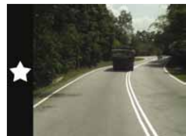
Single carriageway road, narrow paved shoulder, sharp curves, poor roadsides, 90 km/h
