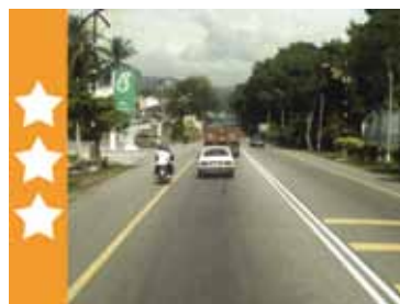
Single carriageway road, wide paved shoulder for motorcycle use, 50 km/h
